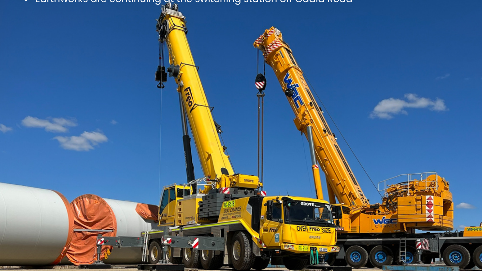
CRANES IN PREPARATION FOR THE CONSTRUCTION OF TURBINE 6
