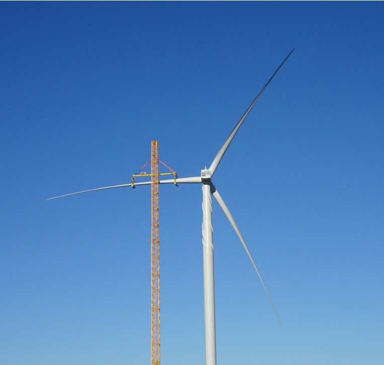
ASSEMBLY OF TURBINES IN COLLECTOR GROUP 3 DURING APRIL 2023
