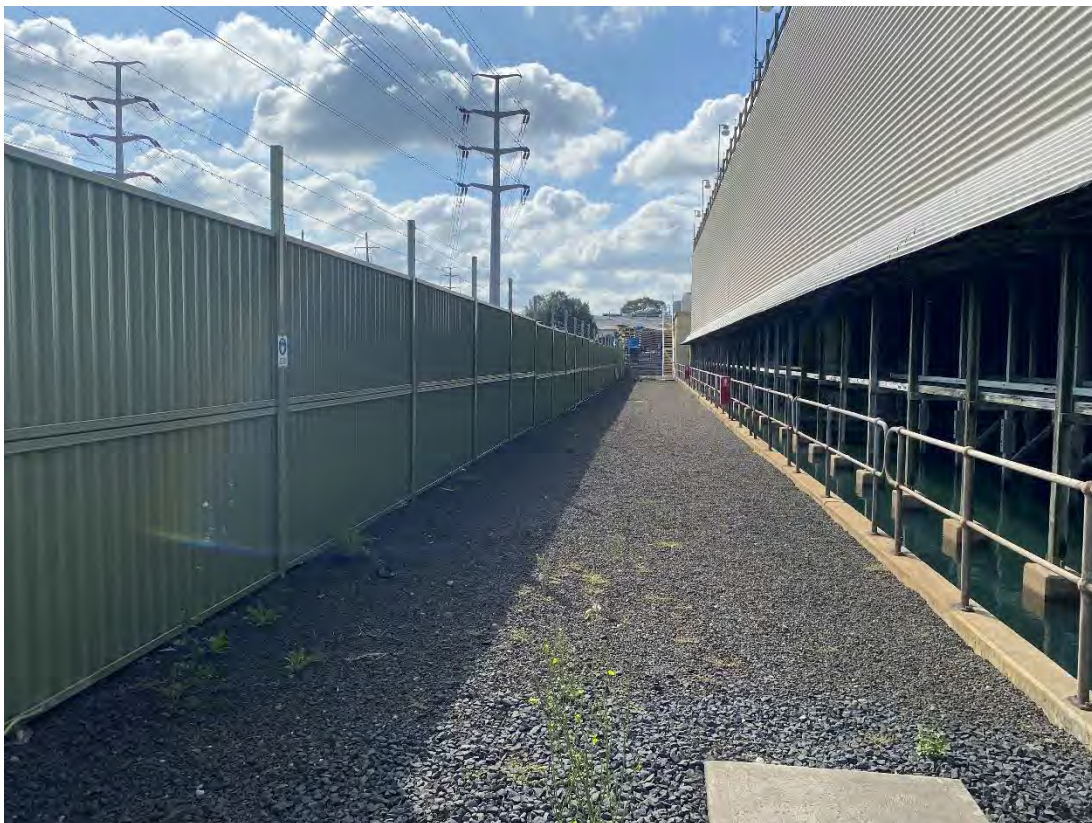
Figure 10 Northern SEF boundary fence and cooling towers
