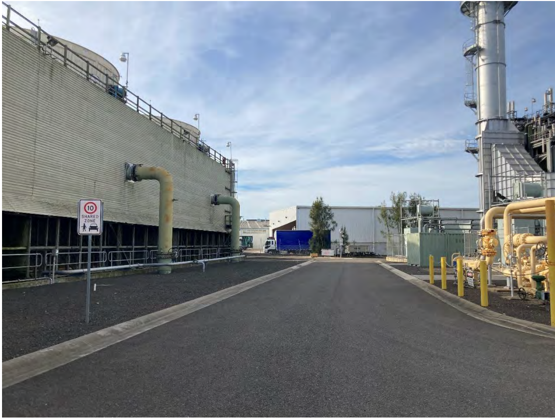
Figure 9 Cooling towers and northern internal road
