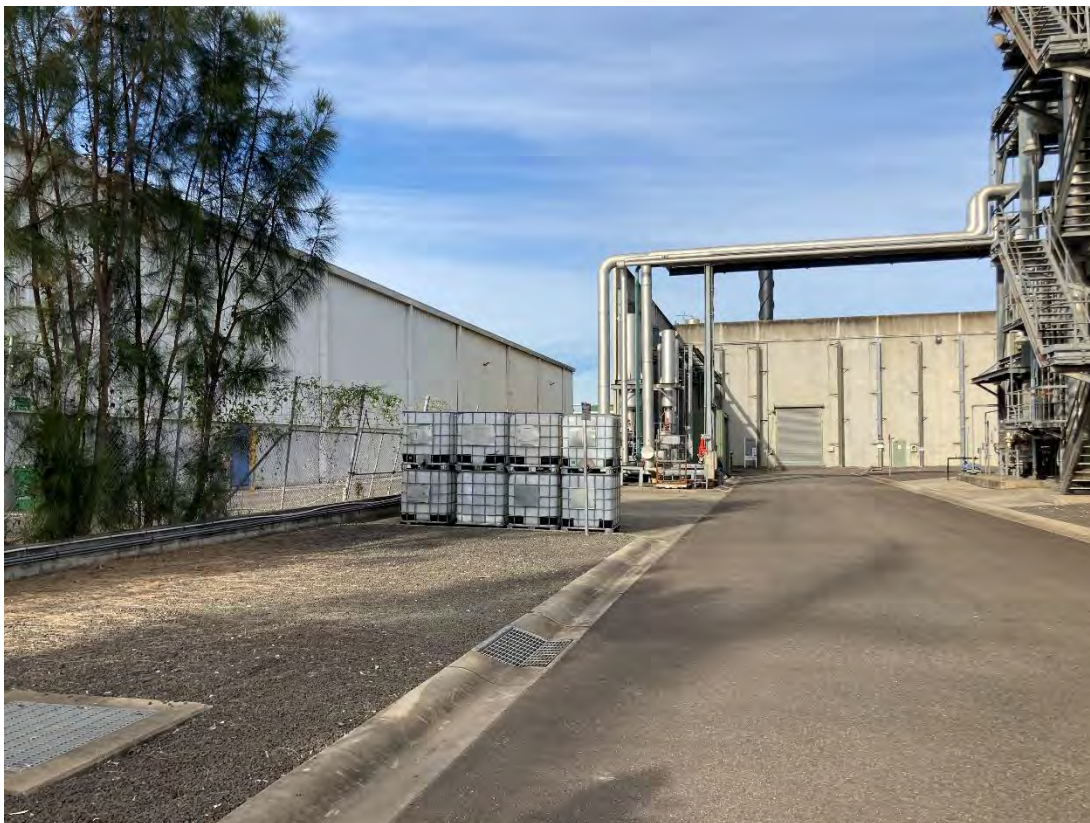
Figure 6 Eastern SEF boundary and eastern internal road
