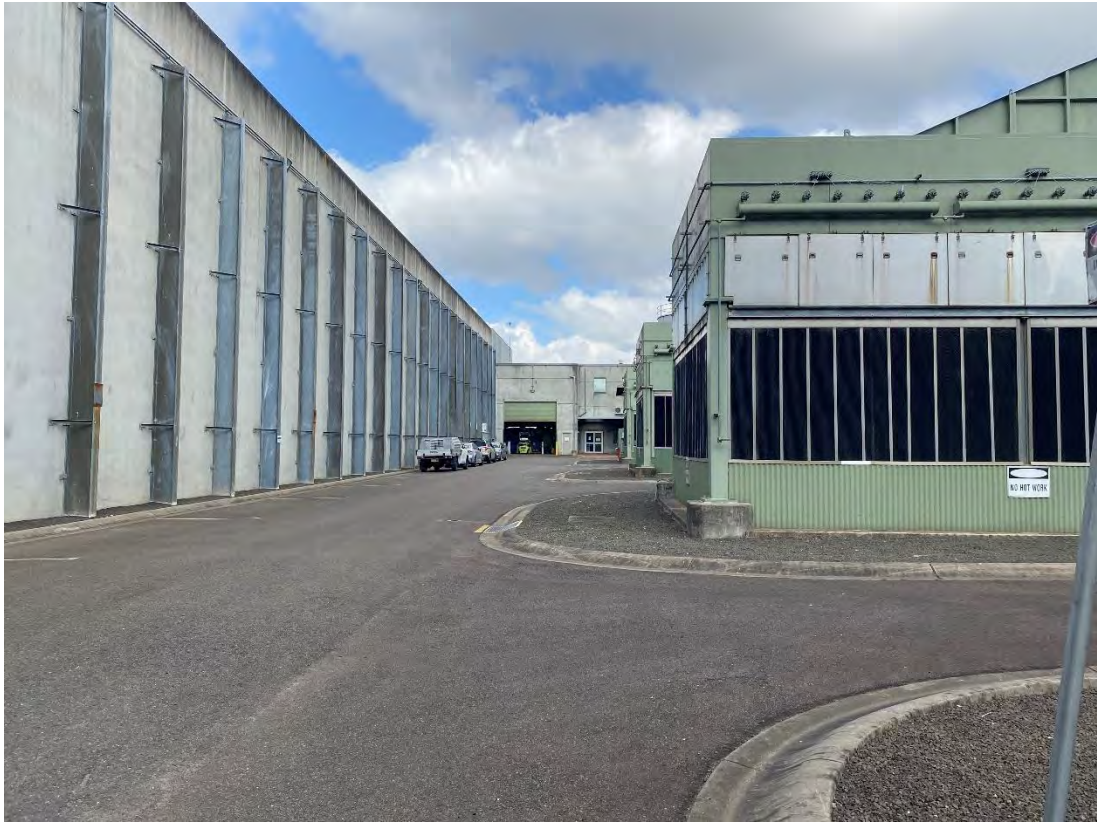
Figure 3 Southern SEF boundary acoustic wall and southern internal road
