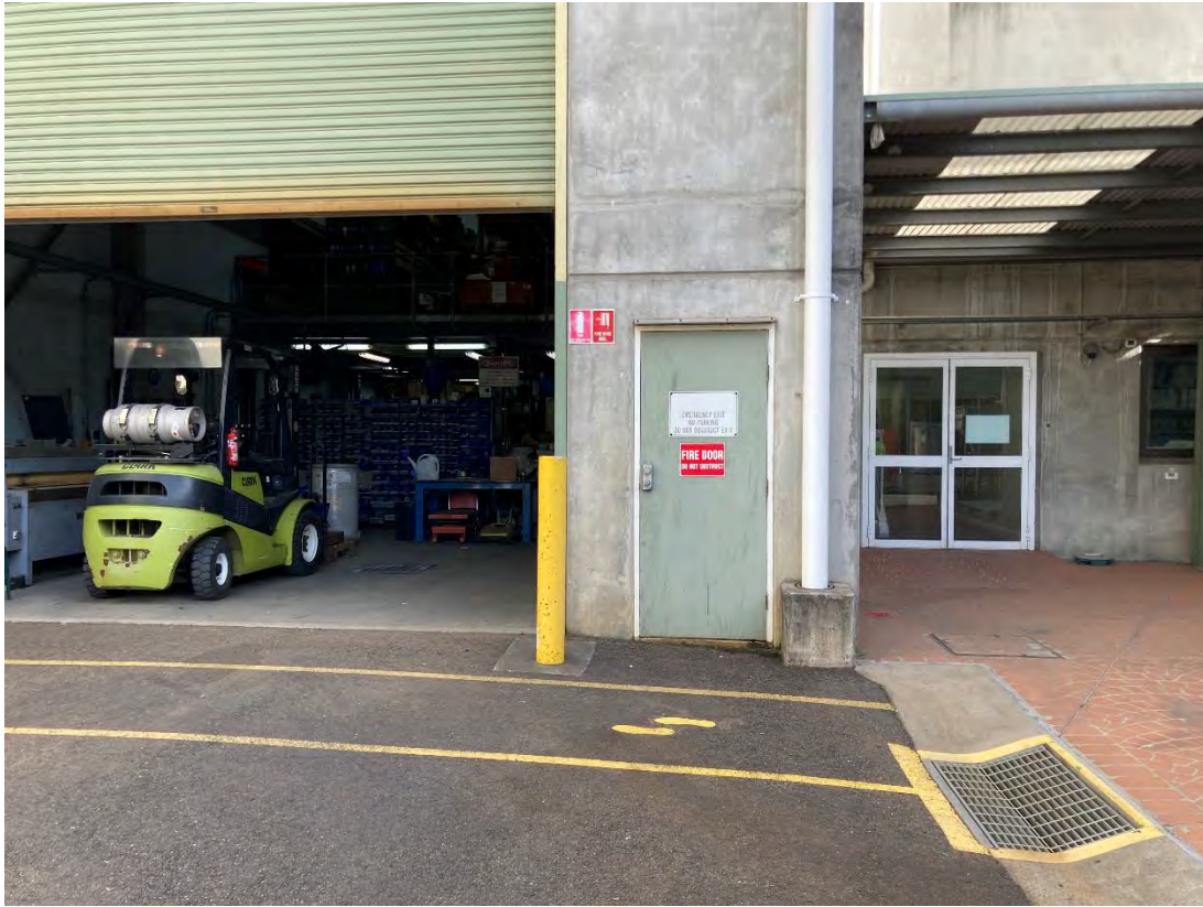
Figure 1 SEF workshop and site office entrance
