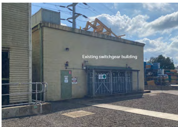
Figure 4-3: Existing switchgear building
